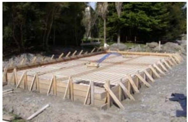
Above and below: The foundations of Orana's Maud Island Frog Habitat prior to the first pre-pour inspection of the concrete foundation. Photos: Orana Wildlife Park.
