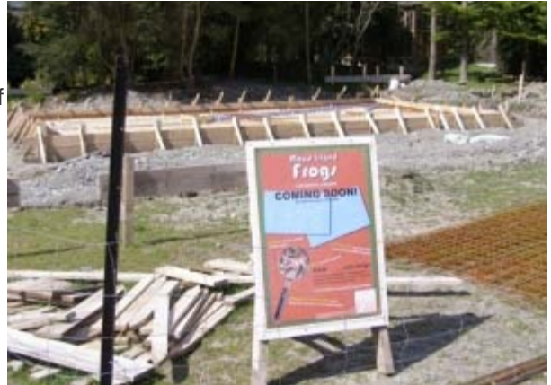
Above and below: The foundations of Orana's Maud Island Frog Habitat prior to the first pre-pour inspection of the concrete foundation. Photos: Orana Wildlife Park.
