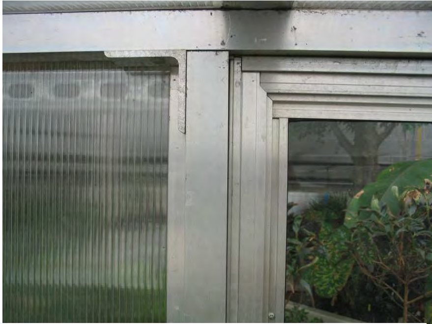
Figure 3. Close-up of the 1 in. (2 cm) aluminum angle pieces holding the 1.5x1.5 in. (3.8x3.8 cm) aluminum tubing and storm door.
