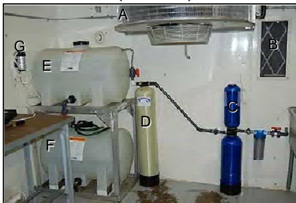
Figure 15. A water filtration assembly for removing chlorine and phosphate . A) Air handling unit; B) Air filter placed over the air intake of the room; C) Pre filter and carbon filter assembly; D) Arsenic/phosphate filter manufactured by BASF and distributed by Aquasana® in Houston, Texas; E) Filtered water reservoir; F) Reconstitution barrel where minerals and salts are added back to the RO water; G) ProMist® mister motor that delivers spray to each of the enclosures in the room. (Photo: J. Pramuk)
