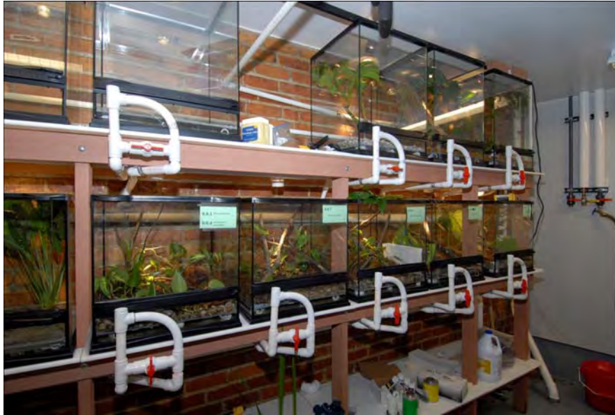
Figure 3. Each tank has its own standpipe overflow created out of “T” and flexible PVC, serviced by a quick-drain valve. All these drains flow into a two-inch common drain pipe created by drilling a hole in the pipe and loosely fitting the \frac{3}{4} -inch drain into the pipe. This prevents siphoning between cages.
