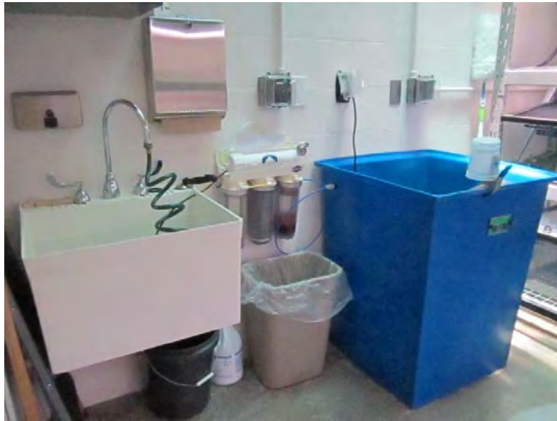
Figure 4. Service area within each quarantine room includes a cabinet, sink, hose, and water filtration/storage vat.
