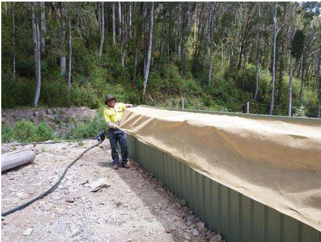
Photo 6. Mesh apron designed to exclude frogs from entering or leaving the field enclosure.
